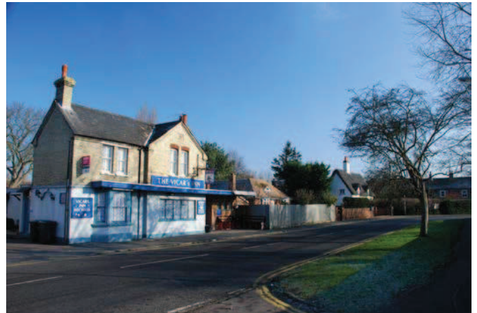
Cream brick Victorian pub (vacant)
